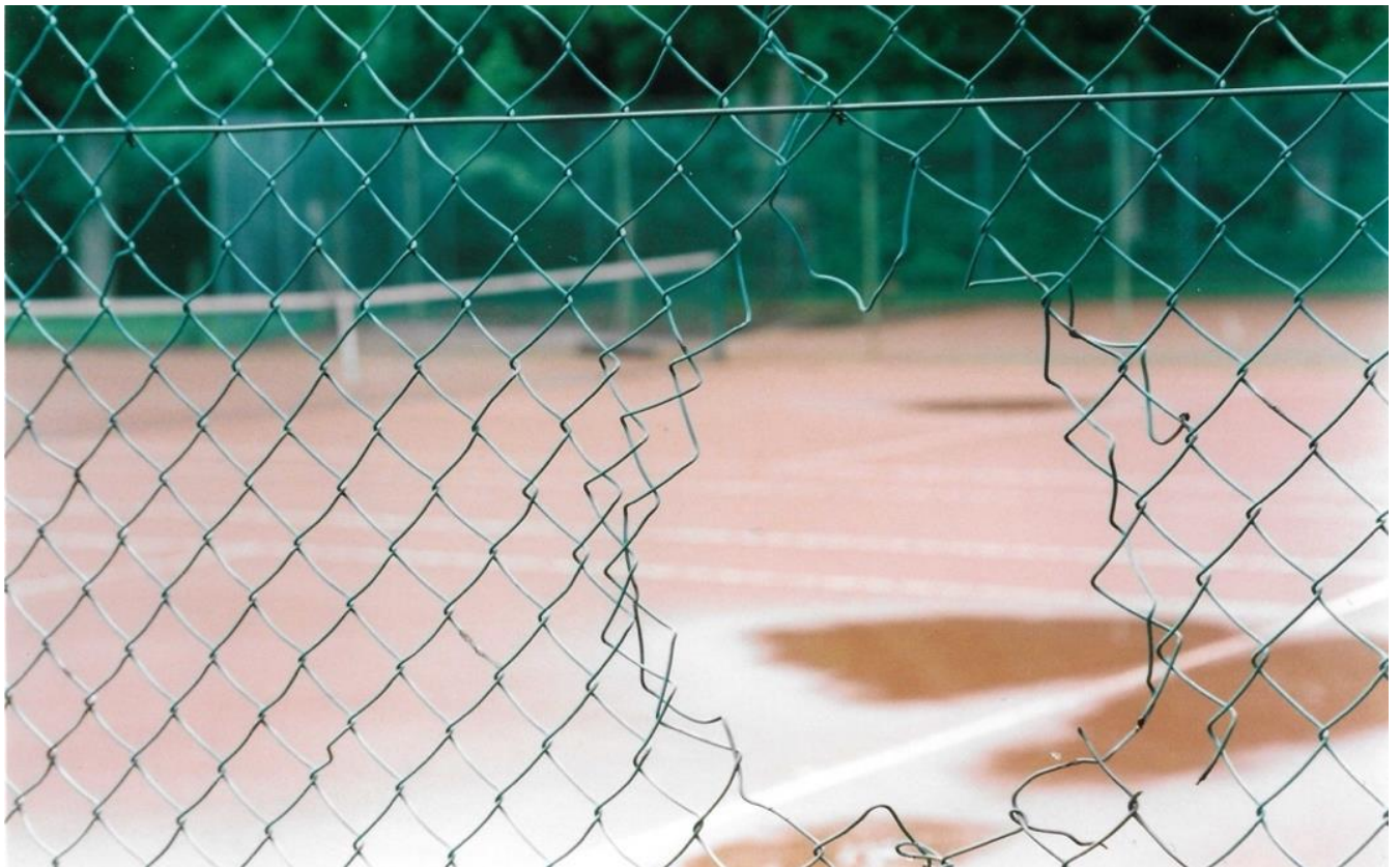
Broken netting on courts one and two
