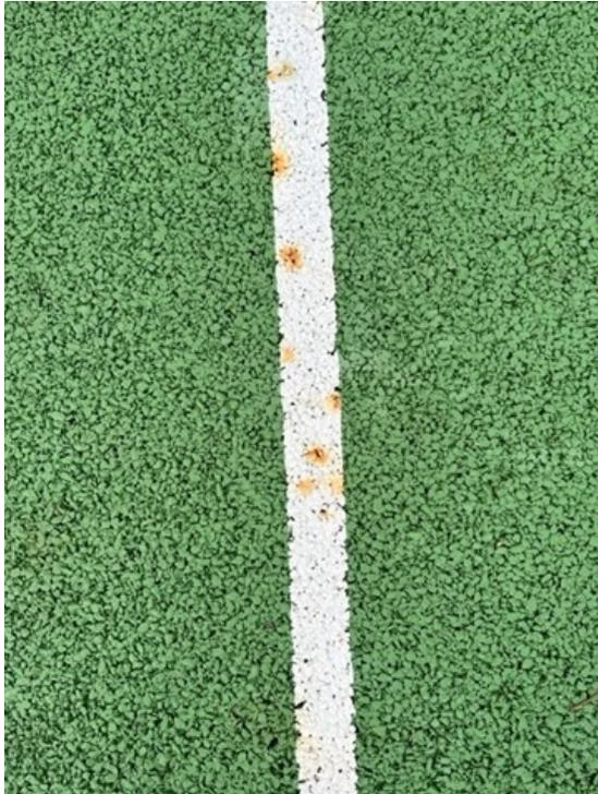
Rust-like brown staining was observed on many of the white line markings; it may also be present on the green court sections, but not be as visible at this time. The staining has been caused by pyrite (iron sulphide) mineral intrusions that are found in many naturally occurring geological rock deposits.
