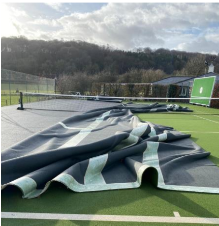
Court 3 storm damage
