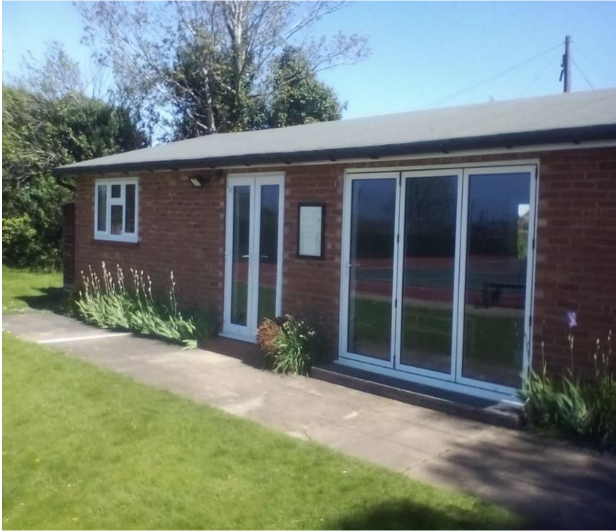
Figure 9. The Clubhouse with refurbished windows and doors
