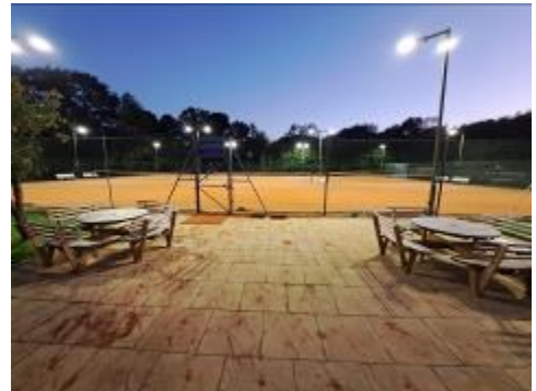
New Flood Lights
